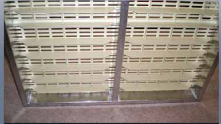
Figure 1. Underside view of Aqua-Dek panels on aluminum frame with 24" on center stringers
